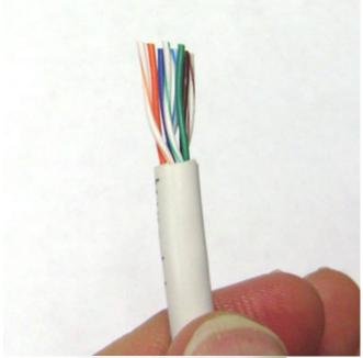
If an insert is unavailable be sure to hold the wires between your thumb and forefinger tightly to keep them in order. Leave about a half inch of the wires exposed and trim the excess length with wire cutters; then, slip on the connector, making sure that the outer jacket is seated in the connector. It may take a few tries to ensure the connectors are in the correct order and are in position for crimping.
